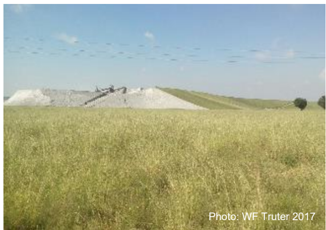
Coal ash dam rehabilitated to a grazing land capability
