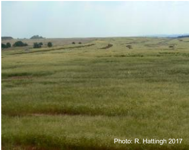
Geomorphically designed flatter outgoing slopes
