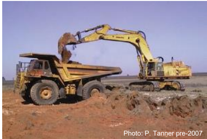
Stripping and replacement using shovel (backhoe) and truck
