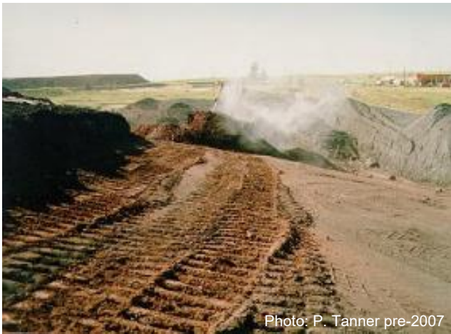
Surface re-shaping in progress
