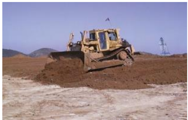
Replaced soil being smoothed by a dozer – the preferred method
